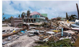
Orient Bay on Saint-Martin after Hurricane Irma.
